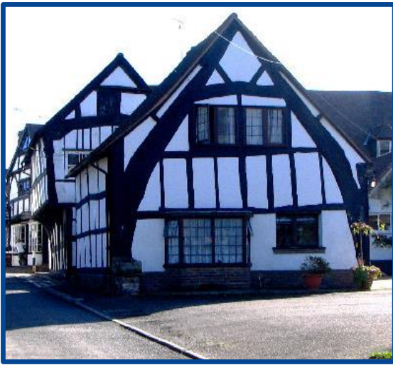
Traditional dowel-connected timber-framed building, England, left and modern timber techniques in the Japanese Pavilion at Hannover Expo (right). Photo credits: Doug Elliot, Jean-Pierre Dalbéra.
